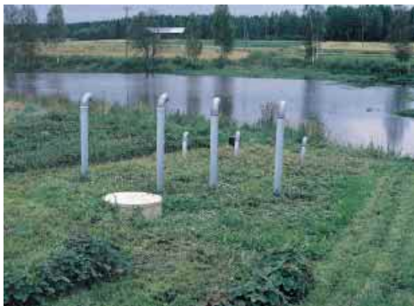
Buried sand filters are presently often used to treat wastewater from single houses.
